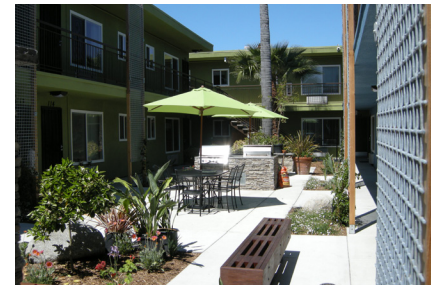
Courtyard after renovation
