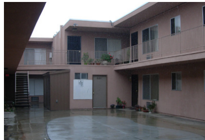
Courtyard before renovation
